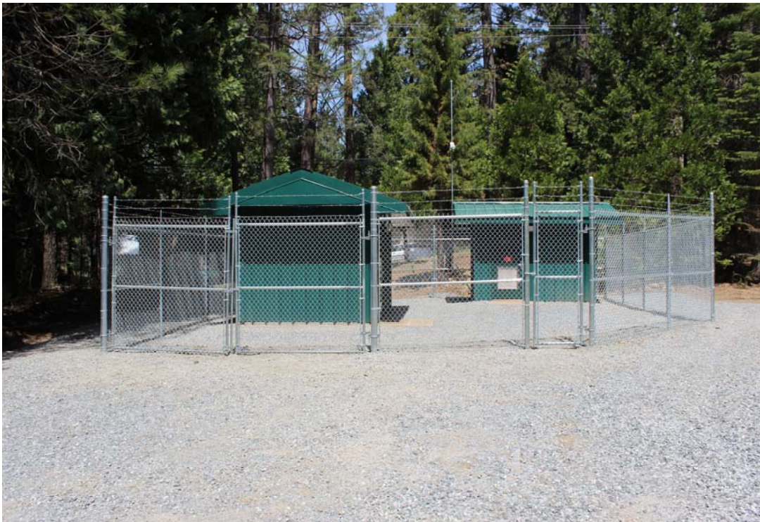
Construction of Well #4 is complete
