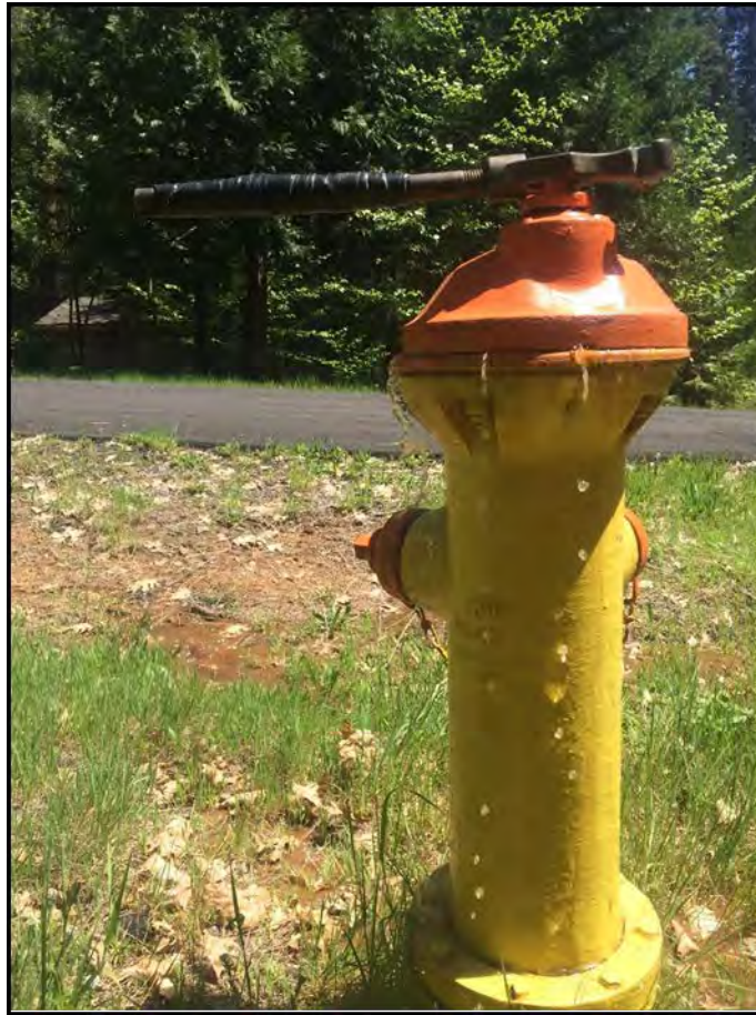
Figure 3.5b Leaking Hydrant
