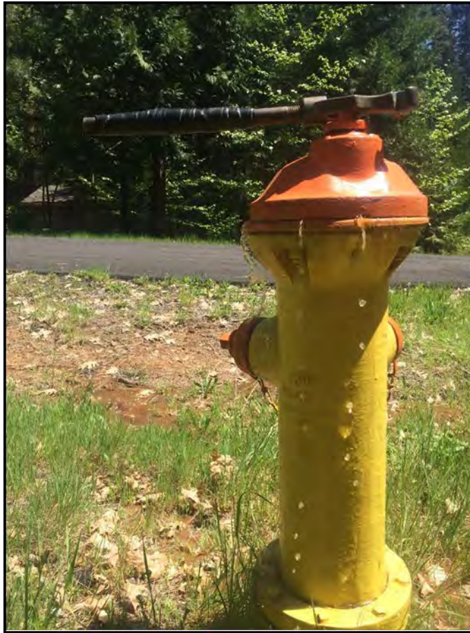
Figure 3.5b Leaking Hydrant
