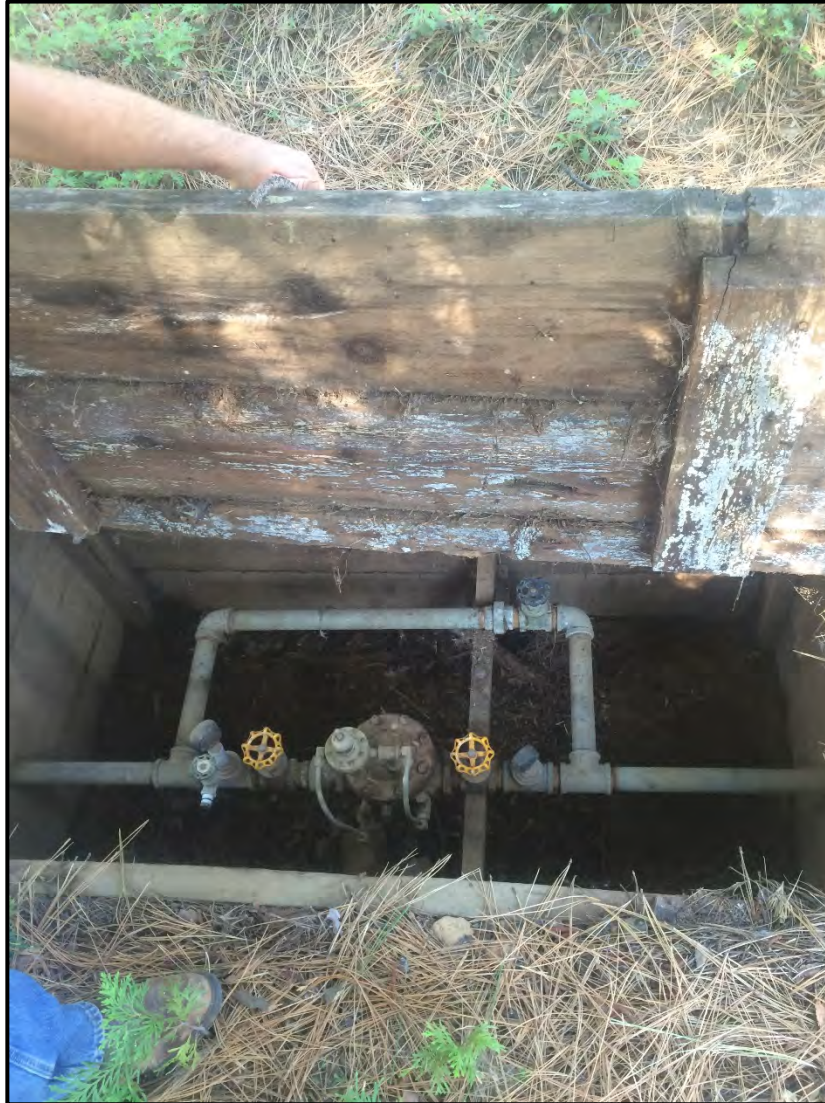
Figure 2.4.5a Deteriorated PRV Station Located on Dorothy Drive
